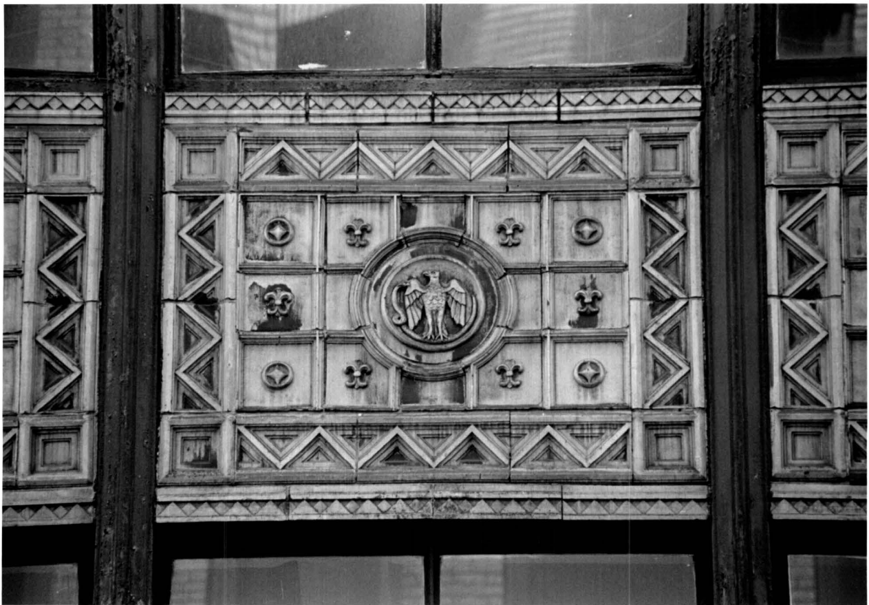
130 West 30 th Street Building, details of terra cotta Photos: Carl Forster
