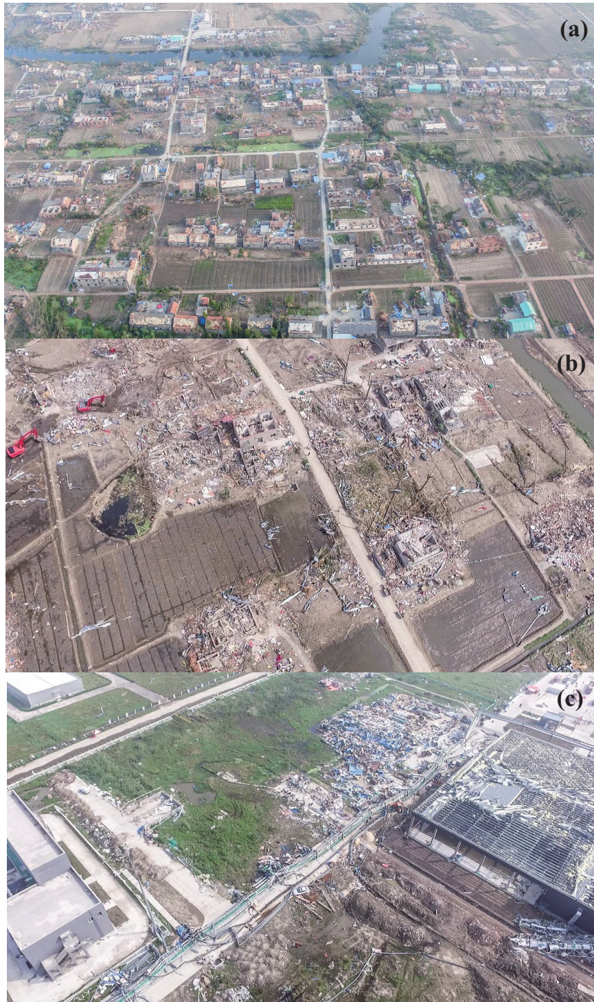
Fig. 1. Aerial survey images showing extensive and severe damage caused by the Funing County, Yancheng City, Jiangsu Province tornado of 23 July 2016.
