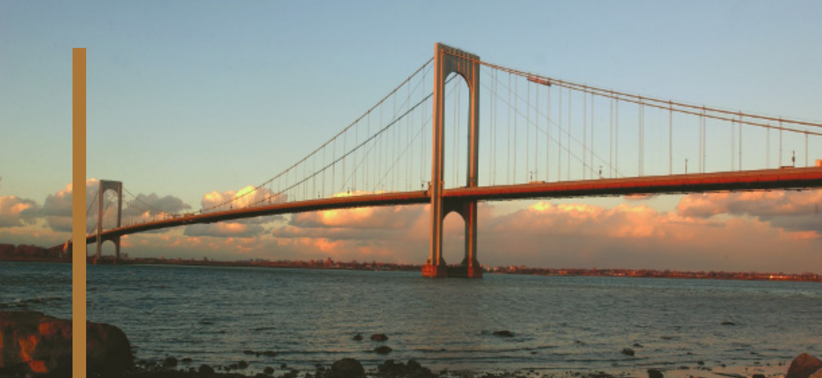
The redecking of the Bronx-Whitestone Bridge was substantially completed in 2006.
