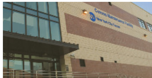
A new maintenance shop and car wash at the Corona Yard, serving the 7 line, was substantially completed in 2006.
