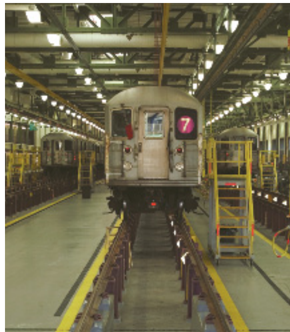
The Corona maintenance facility incorporates sustainable design features.
