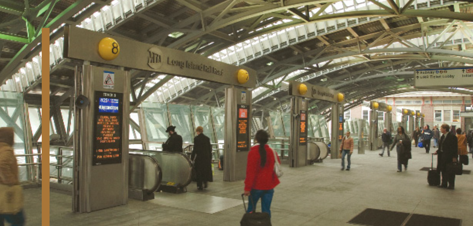
The rehabilitated mezzanine at Jamaica provides access to all LIRR tracks and links to the subway and AirTrain JFK.
