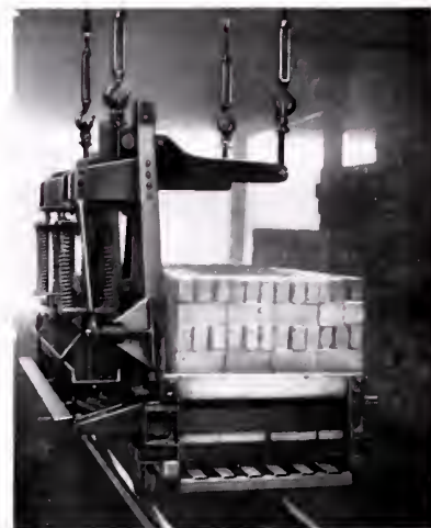
Setting Machine With Load Ready to Lift
