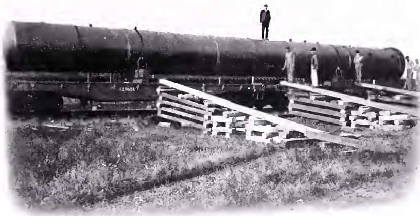
View of Hardening Cylinders at Destination Preparatory to Unloading
