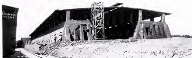
Haigh Continuous Kiln, Showing Coal Elevator 66 Chambers, Three Fires
