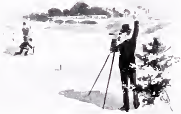
Surveying the grounds and laying out buildings.
