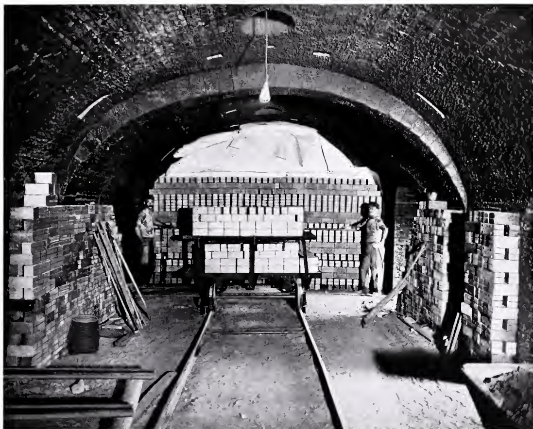
Figure 3, Interior of Haigh Kiln Showing Setting
