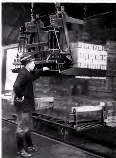
Setting Machine Raising the Load
