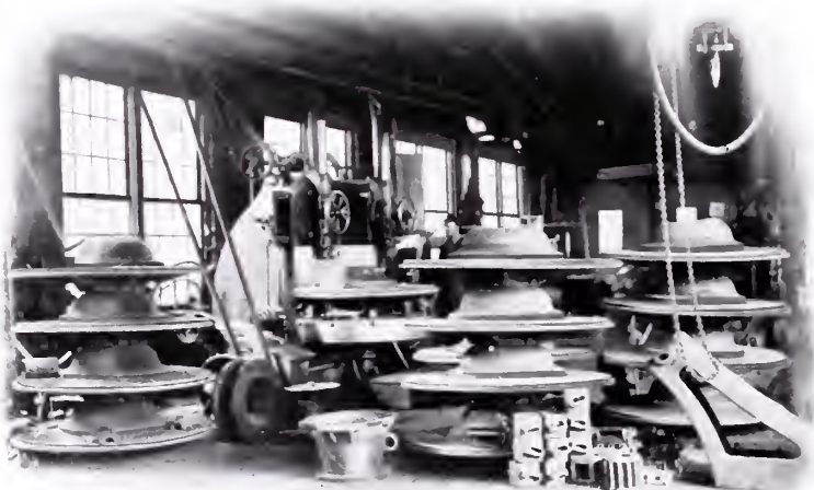
Machining Dry Pan Bottoms — Bringing Through 18 Pans at a Time
