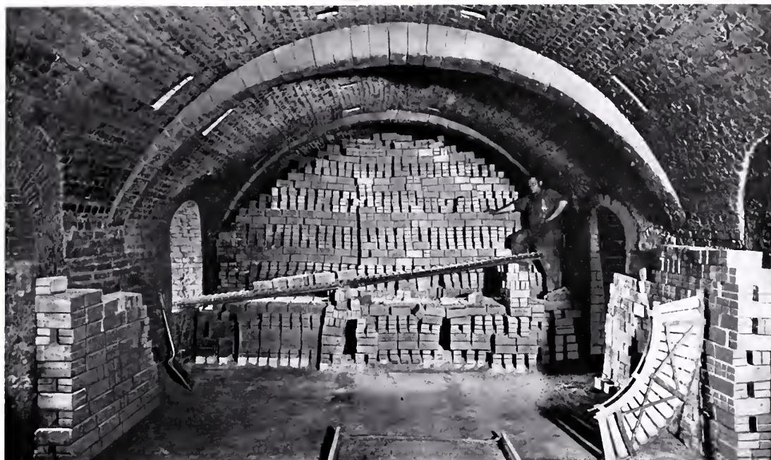
Interior of Kiln Showing Method of Unloading Burned Paving Blocks by Gravity Carriers Also a Good View of the "Drop Arch"
