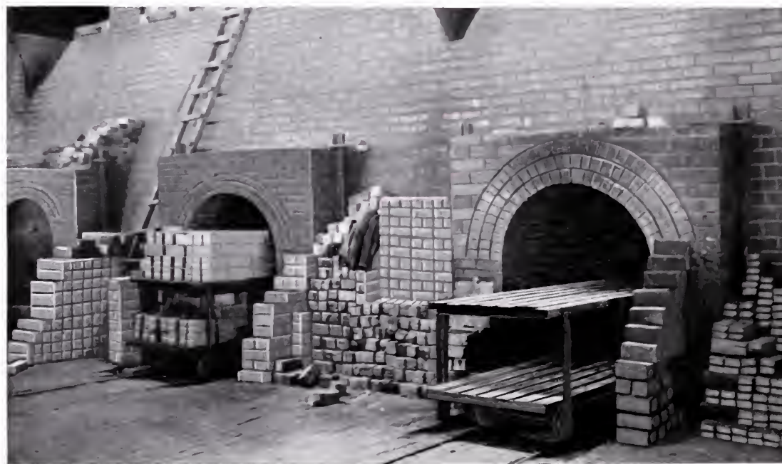
Putting Dry Brick into Kiln and Withdrawing Empty Cars
