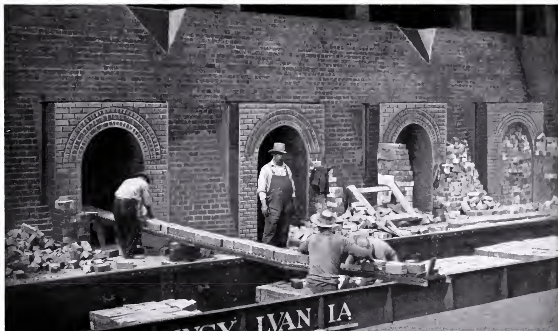
Loading Paving Blocks from Kiln to Cars with Gravity Carriers
