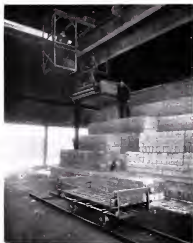
Setting Load of Brick on Top Bench of Kiln. Note Evenness of Brick on Under Side of Load
