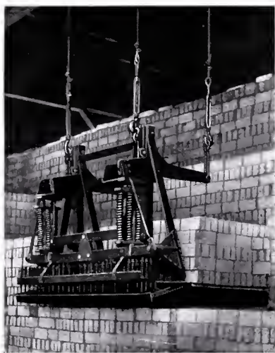
Setting Load of Brick on Third Bench of Kiln
