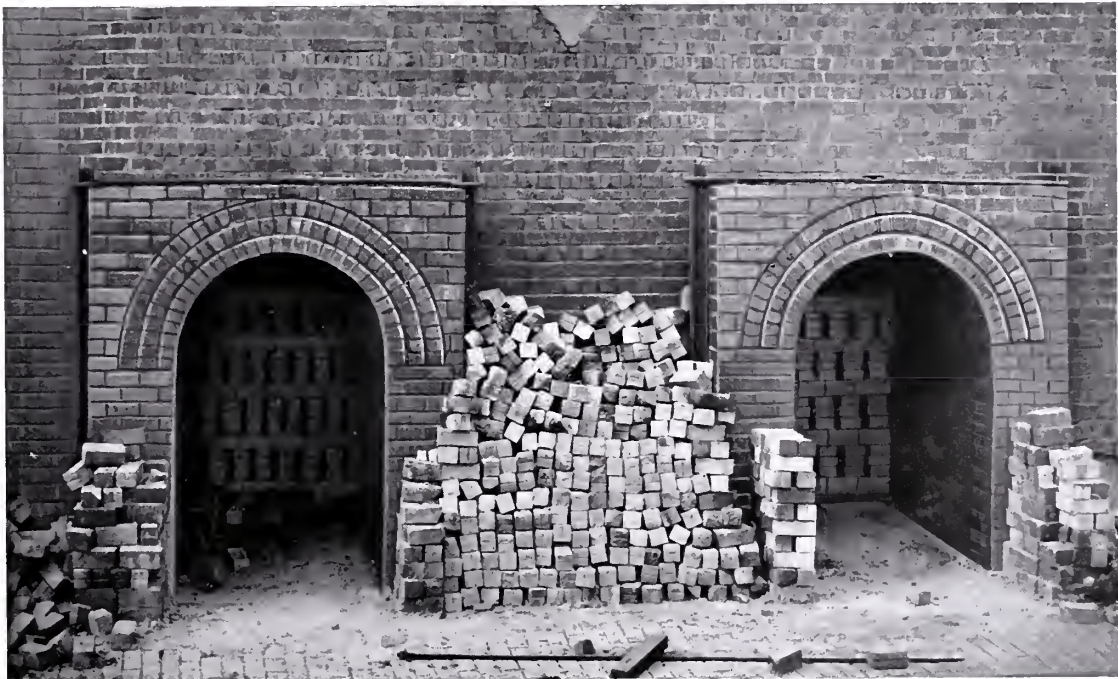
Kiln Doors Just Opened with Burned Brick in View
