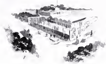
Erecting the Buildings.
