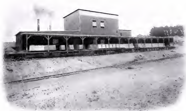
View of Sand-Lime Brick Plants
