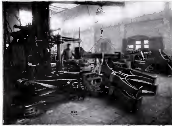
Machining Pan Frames to Make Secure Joints
