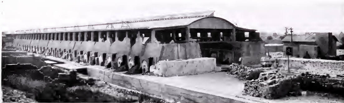
110 Chamber Haigh Continuous Kiln. Five Fires
