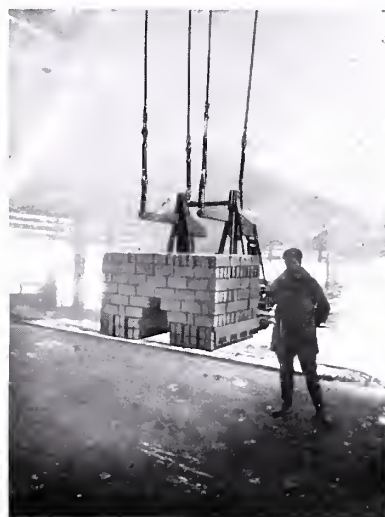
Setting Machine Raising the Arch Unit Note Space Between Bottom Row of Bricks for Fingers to Enter
