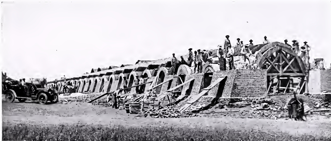
Showing Kiln Under Construction
