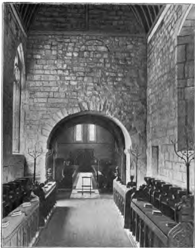
S. PAUL'S CHURCH, JARROW, LOOKING WEST.
