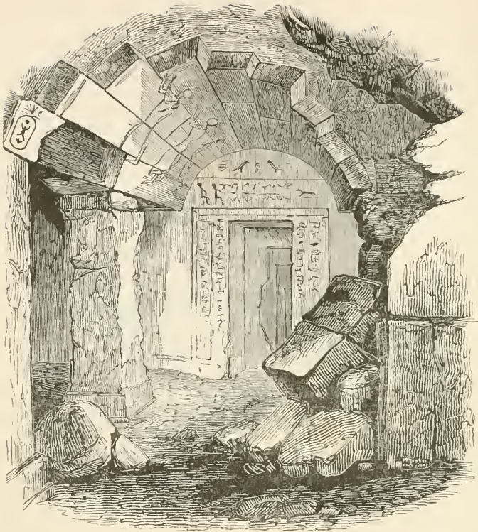
VIGNETTE I. — Tomb at Saqqara, arched with stone, of the time of Psammatichus I., whose name occurs on the roof to the left, and other places.
