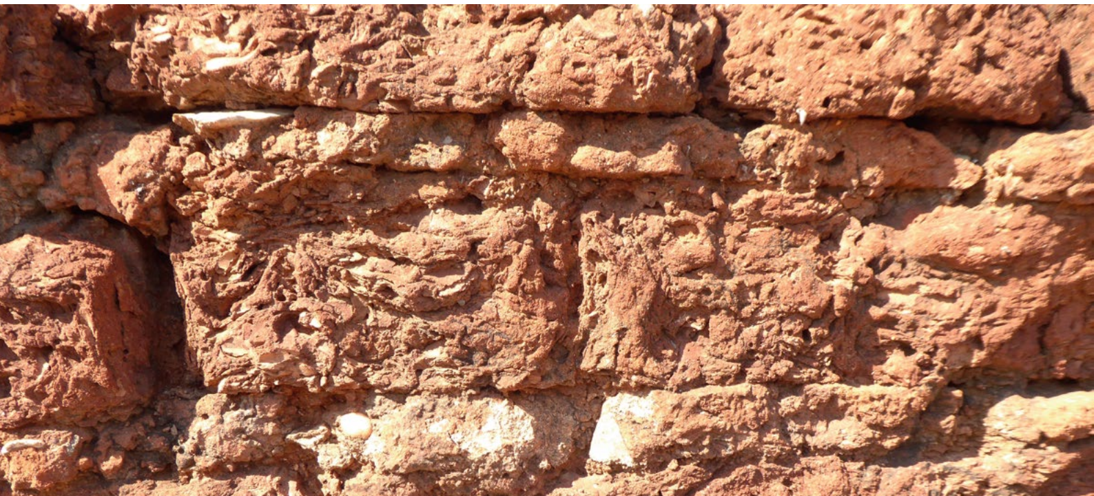
Mud brick wall in the Late Minoan Palace of Malia, Crete (Greece; photo: F. Knoll 2019).
