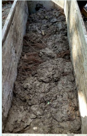
Lattes, Hérault (France), experimental workshop. Constructing a wall by packing cob layers into the wooden frame, separated by branches of heather (photos: C.-A. de Chazelles 2010).
