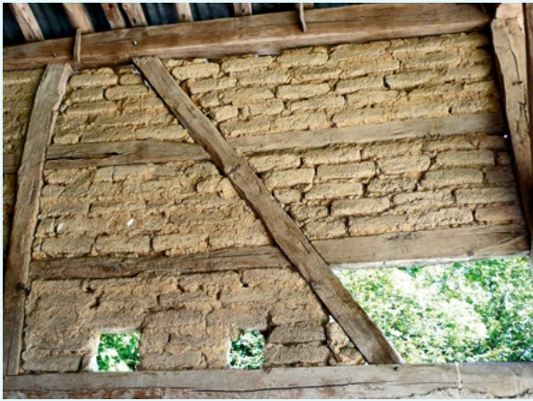
Top: Detail of a half-timbered barn. The panels were filled with adobe. Moivre, Marne (France; photo: C.-A. de Chazelles 2009). Bottom: House with half-timbered upper storey in Mötzlich, Saxony-Anhalt (Germany), built in 1758. The timber framing was filled with mud bricks, whereas other parts were filled with vertical rods (photo: F. Knoll 2017).
