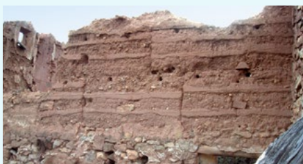
Top: Pisé wall of a ruinous building at Hortichuela, Valencia (Spain; photo: M. Pastor Quiles 2015). Left: Pisé-built dwelling at Steigra, Saxony-Anhalt (Germany). In this region, the single rammed layers are divided by roof tile fragments (photo: F. Knoll 2015).
