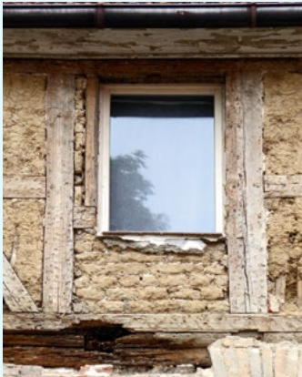
Top: Detail of a half-timbered barn. The panels were filled with adobe. Moivre, Marne (France; photo: C.-A. de Chazelles 2009). Bottom: House with half-timbered upper storey in Mötzlich, Saxony-Anhalt (Germany), built in 1758. The timber framing was filled with mud bricks, whereas other parts were filled with vertical rods (photo: F. Knoll 2017).
