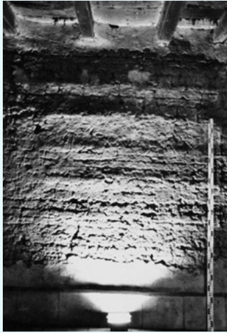
Farm at En Vidalot, Beaumont-de-Lomagne, Tarn-et-Garonne (France; 17 th century AD), inner side of the wall. The imprints of the wooden formwork are still visible, as well as the single cob units used to erect the wall (Klein 2003, 422 Fig. 7).
