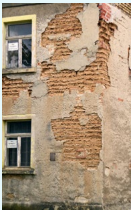
Top: Pisé wall of a ruinous building at Hortichuela, Valencia (Spain; photo: M. Pastor Quiles 2015). Left: Pisé-built dwelling at Steigra, Saxony-Anhalt (Germany). In this region, the single rammed layers are divided by roof tile fragments (photo: F. Knoll 2015).
