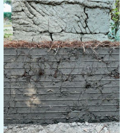
Lattes, Hérault (France), experimental workshop. Constructing a wall by packing cob layers into the wooden frame, separated by branches of heather (photos: C.-A. de Chazelles 2010).
