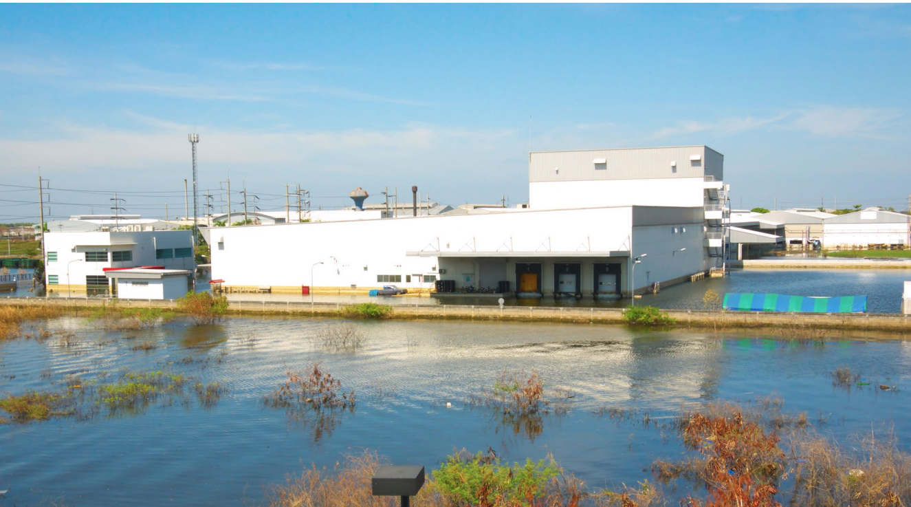
Water flood in industrial estate
