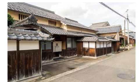
This hotel in the post town was renovated from a former merchant's residence
