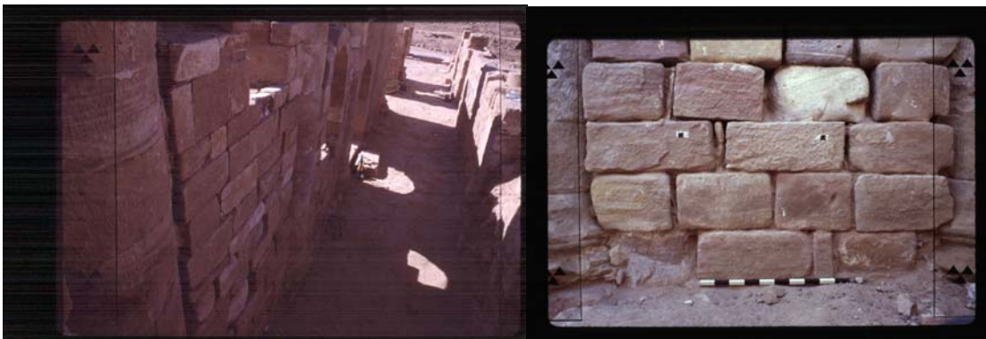
Figure 53 Shows the West Corridor of the Great Temple. This region is difficult to document because it's not possible to get clear shots of the whole elevation. In this instance it was necessary to take close-range shots of the various sections to ensure that the elevations could be reconstructed with wall detail.
