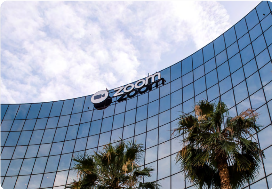
Left: Looking above the entrance of Zoom HQ in San Jose, California
