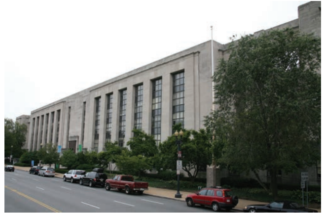
Washington, D.C. VOA Headquarters is in the Wilbur J. Cohen Building.
