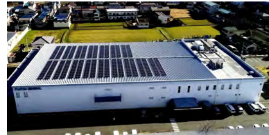
Solar panels on the roof of our Matsubara Office (operation from January 2024)
