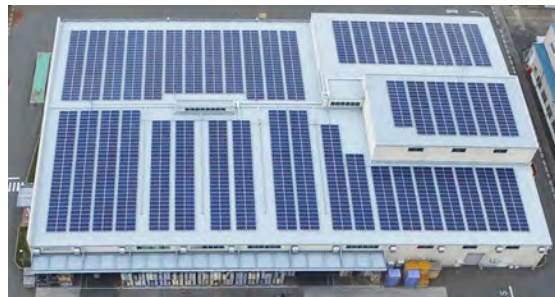
Solar panels (Operation from December 2017)
