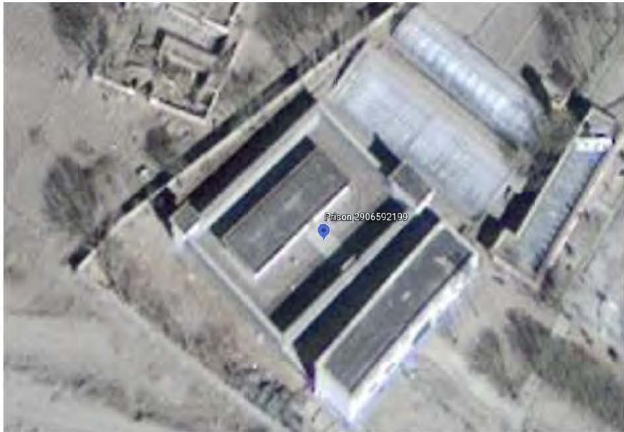
Figure 113 - Langkazi County Detention Center 2906592199
