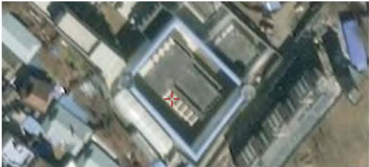
Figure 72 - Dazi County Detention Center
