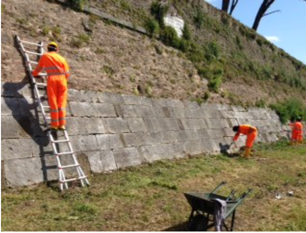
Cleaning the walls
