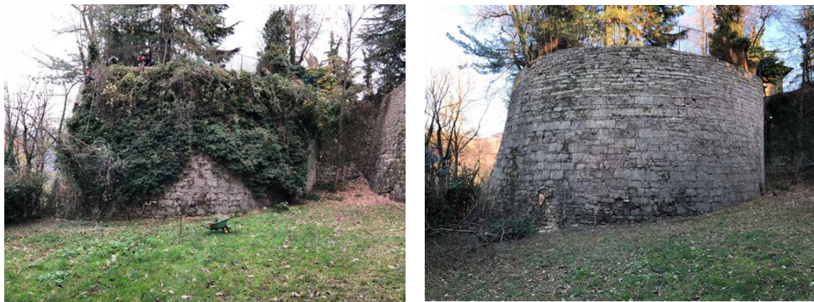
Figure 3 - Vegetation clearing in Section D15 (before and after)
