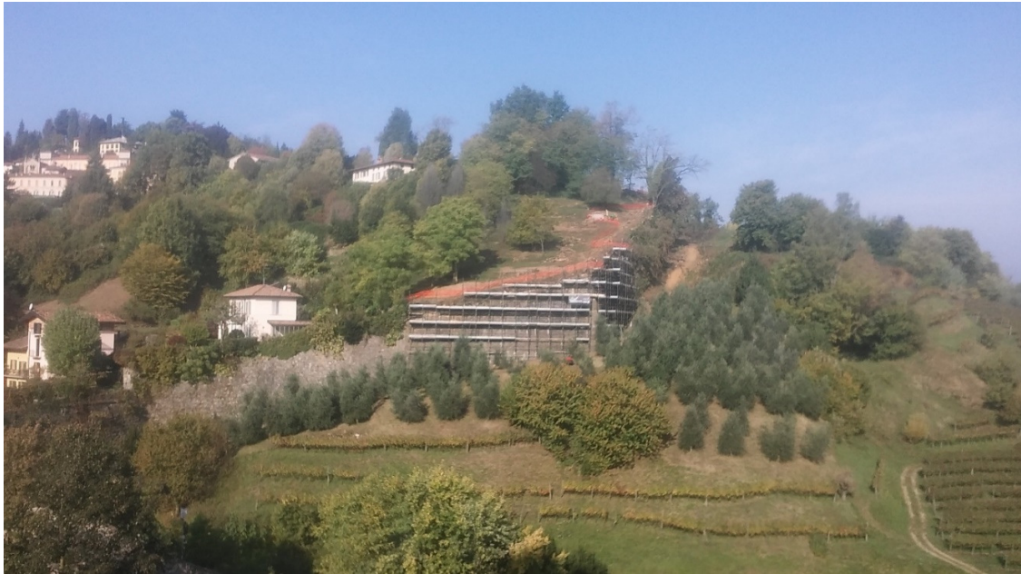
Figure 4 - Clearing and restoration work on the Valverde Rampart
