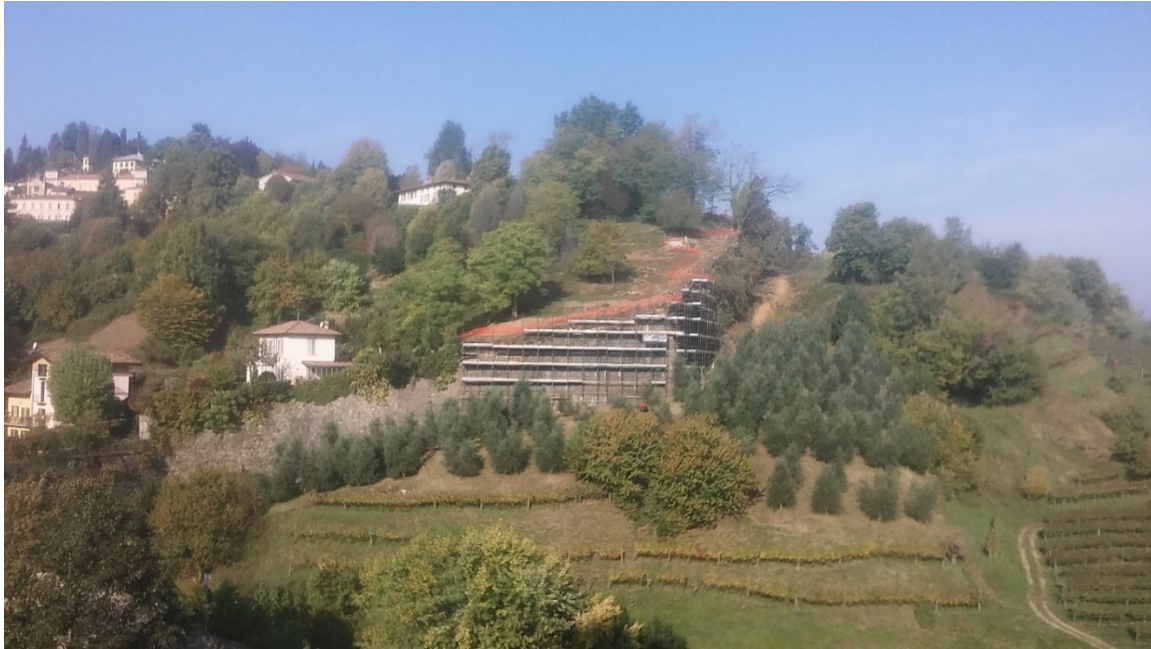
Figure 4 - Clearing and restoration work on the Valverde Rampart
