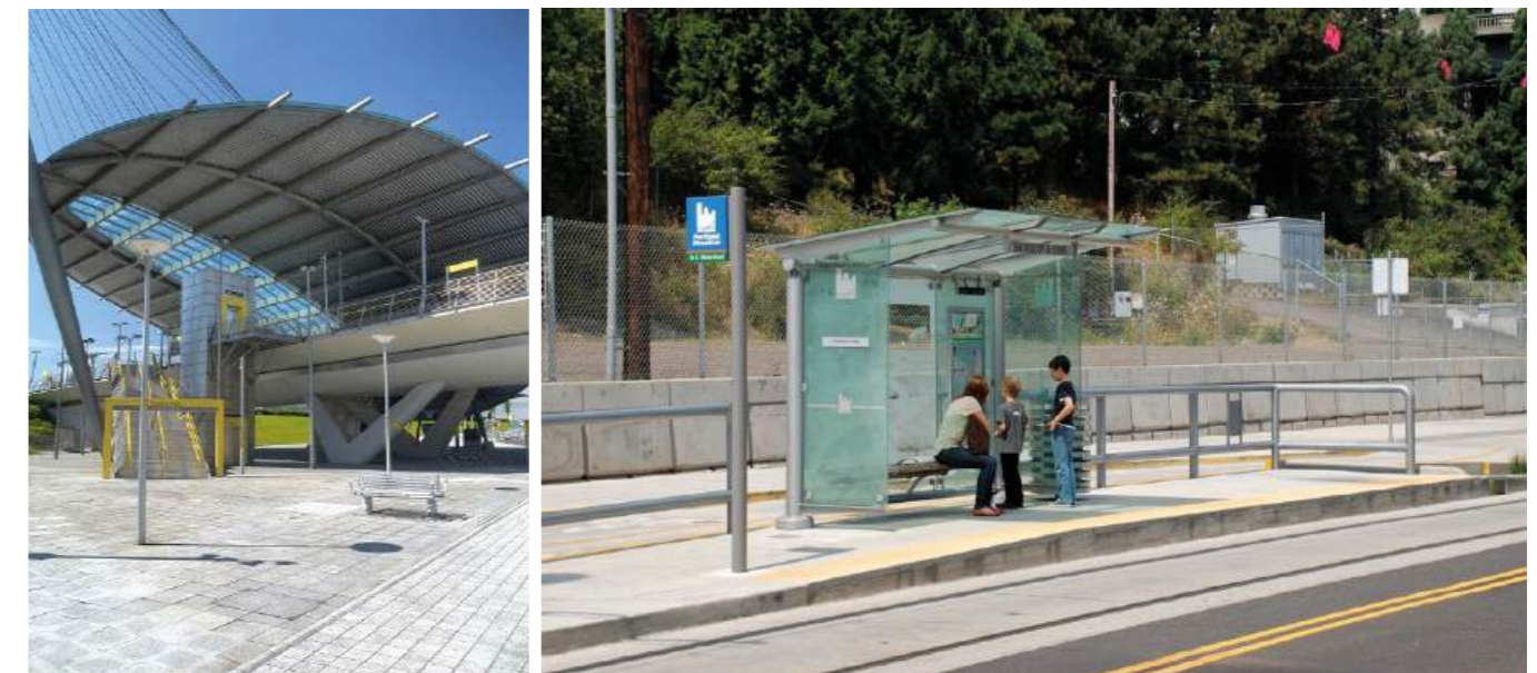
The architecturally interesting, but very costly, Central Park Station on the Manchester Metrolink (left: source David Dixon, wikimedia ) versus the standardised, inexpensive, and easy to use Moody and Gibbs stop of the Portland Streetcar (right: source: Steve Morgan, wikimedia ).
