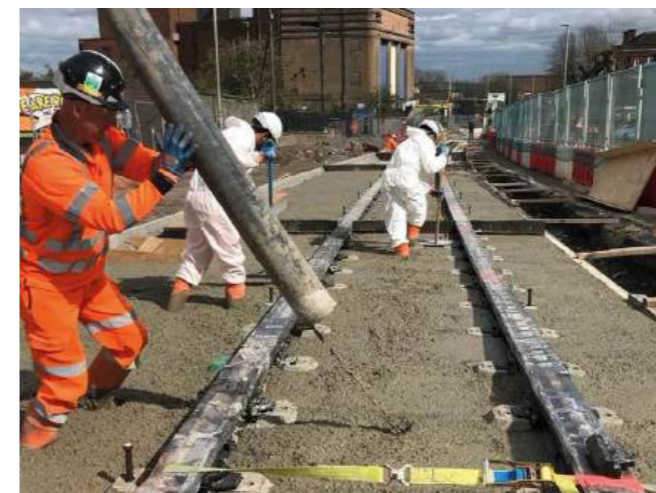
Left: workers completing the track bed on the West Midlands Metro, which is deeper than the European norms, requiring significant concrete (source: Midlands Metro Alliance). Right: the shallower and simpler track bed of Vienna's trams (source: courtesy of Amey Ltd).
