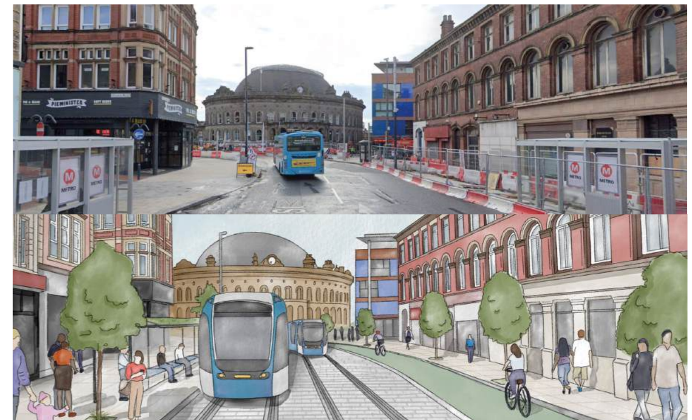
Duncan Street today and in 2035 with a tram and improved public realm.
