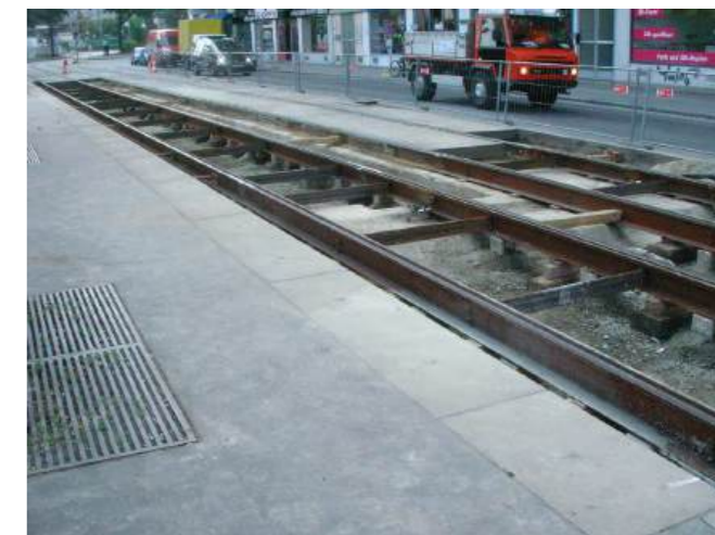
Left: workers completing the track bed on the West Midlands Metro, which is deeper than the European norms, requiring significant concrete (source: Midlands Metro Alliance). Right: the shallower and simpler track bed of Vienna's trams (source: courtesy of Amey Ltd).
