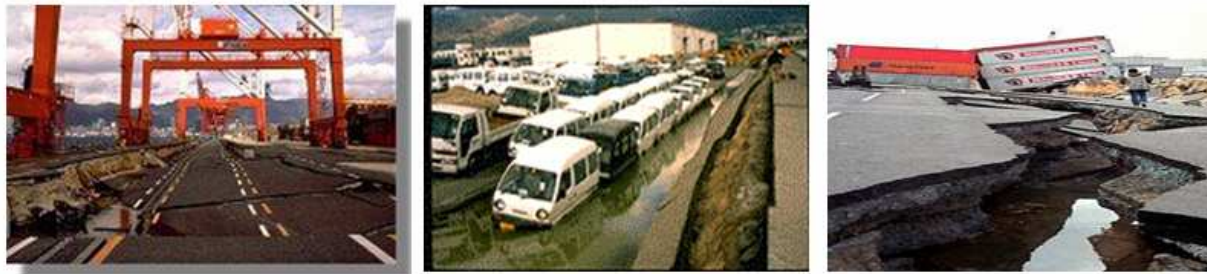
Fig. 1 Results of liquefaction of backfill behind quay wall following Kobe earthquake
