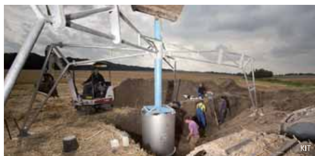
Lysimeter installation for analysis of precipitation, evaporation, variation of water storage, and seepage water formation.
