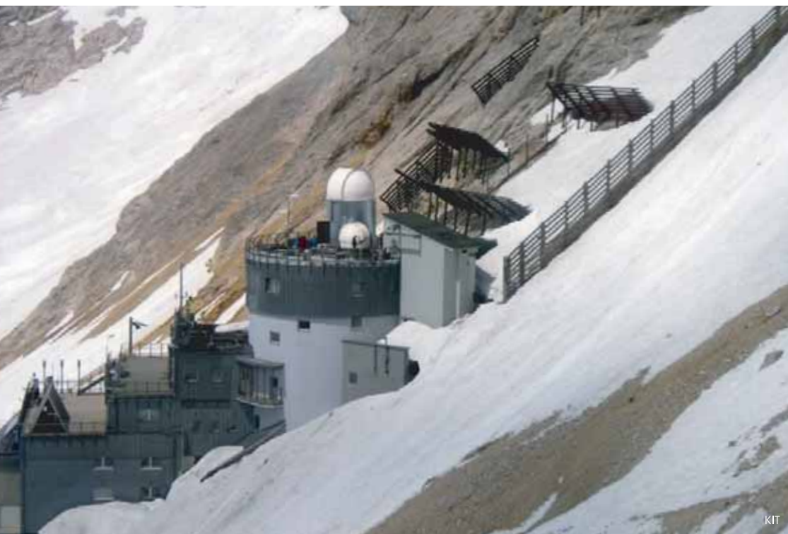
KIT performs lidar vertical soundings of water vapor above the research station Schneefernerhaus.
