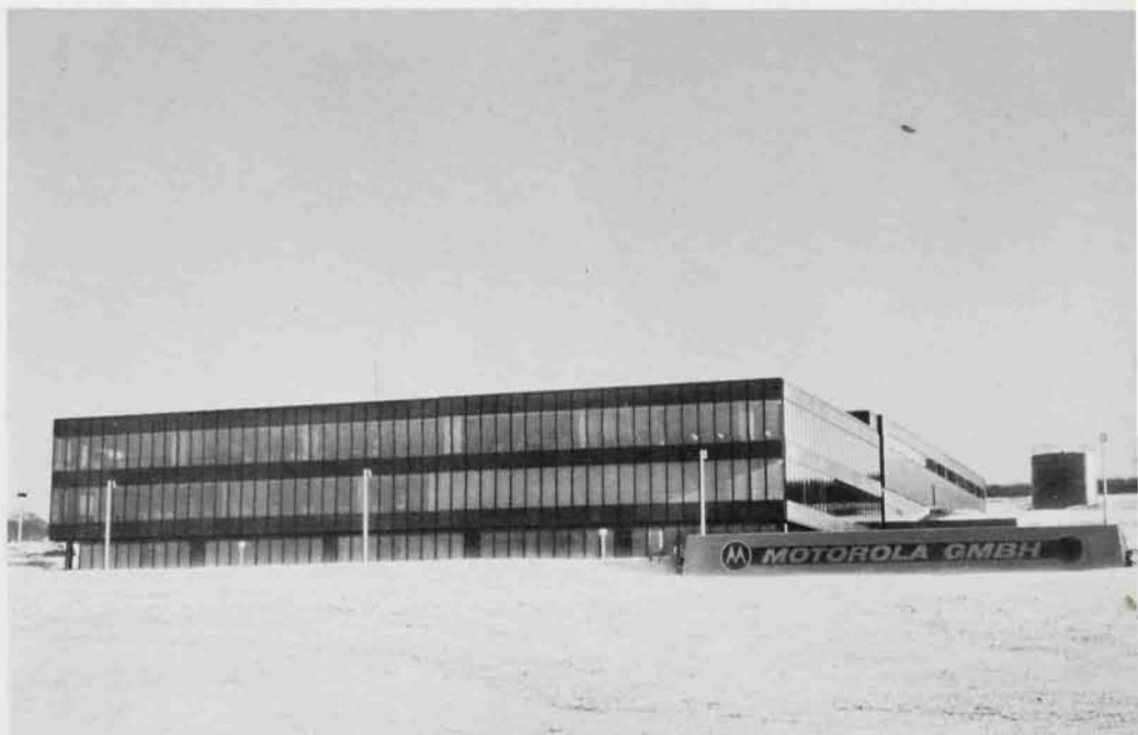
The new European headquarters for the Communications International Division at Taunusstein was formally dedicated in 1975.
