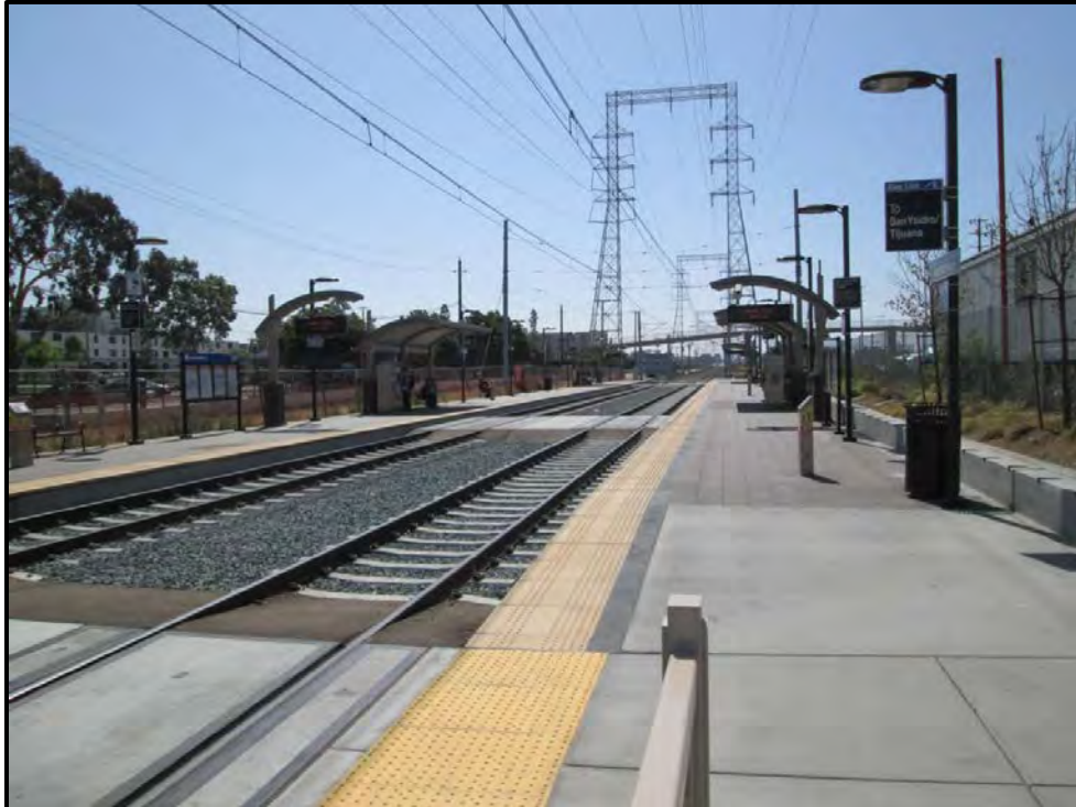
Figure 5: MTS Blue Line Pacific Fleet Station. View looking south.
