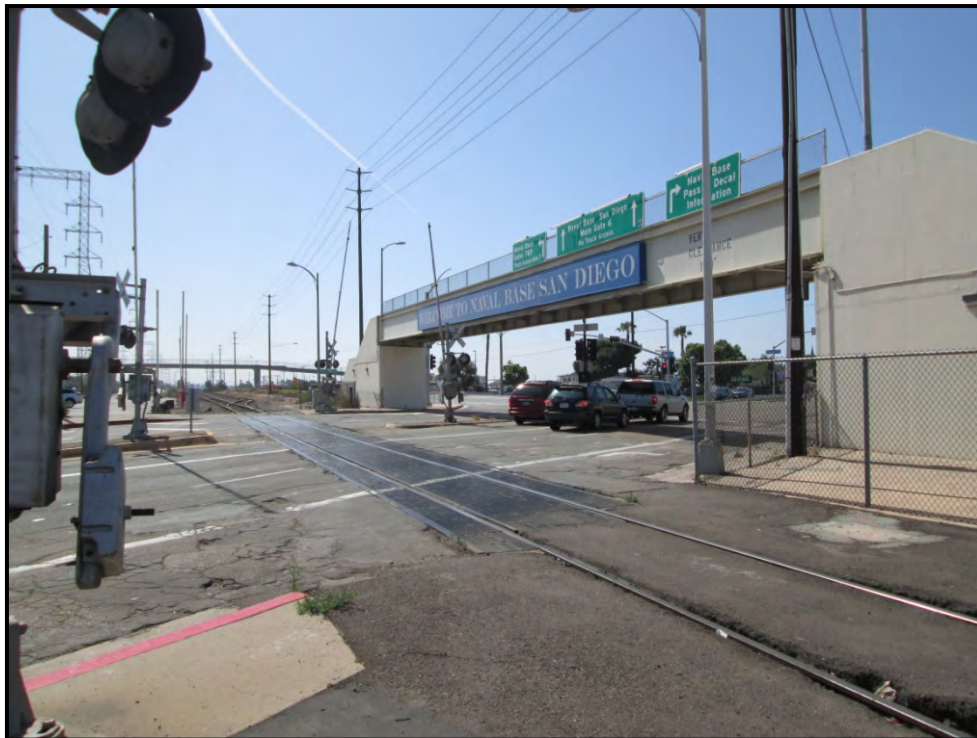
View of the ATSF rail lines in the ROW. View looking south.
