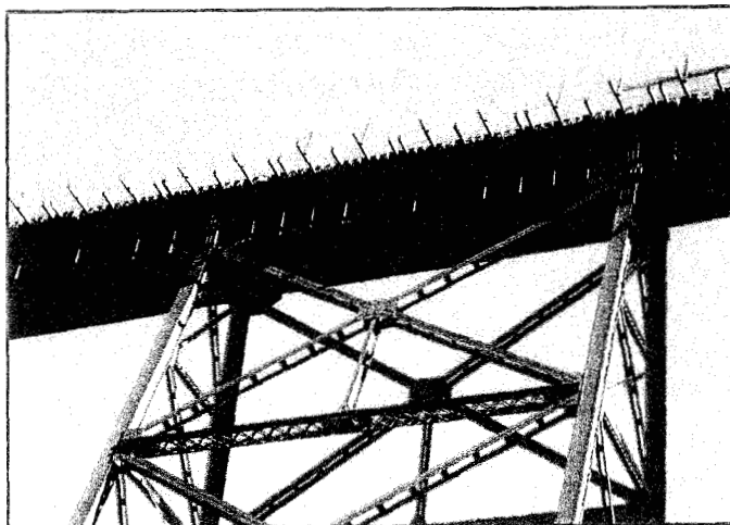
Upper portion of trestle looking east.
