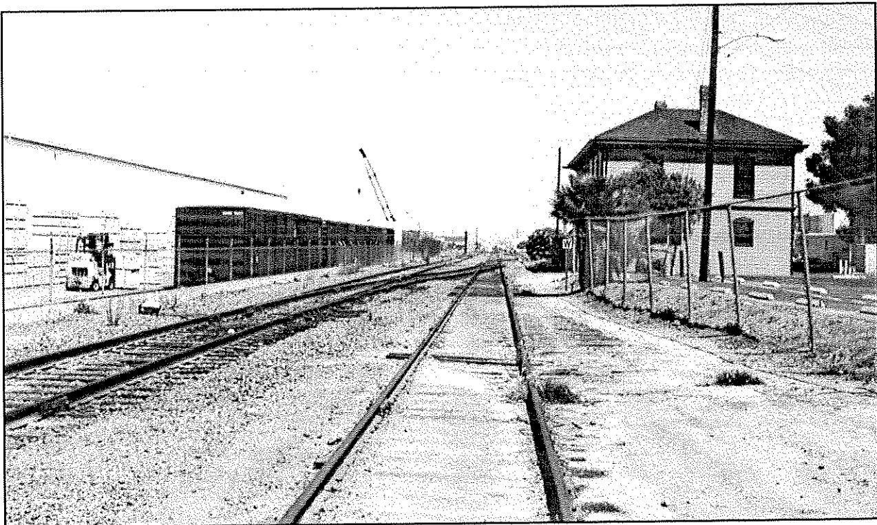
Abandoned segment of old railroad near the National City depot. (View to the north)
