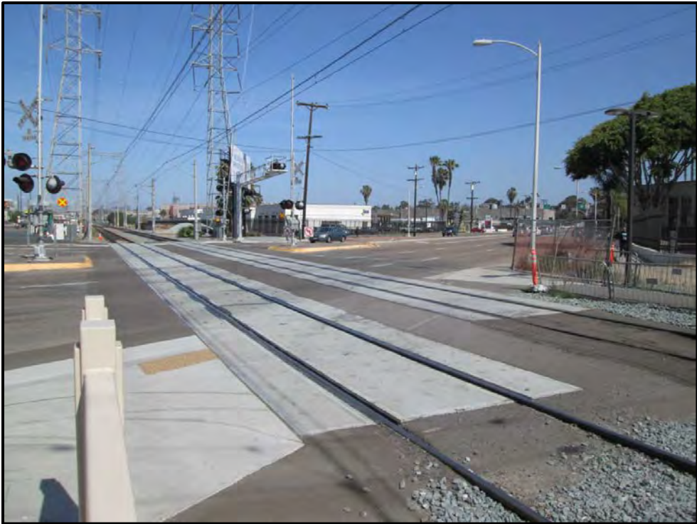
Figure 4: MTS Blue Line Trolley rails and overhead power lines intersecting with 32 nd Street. View looking north.
