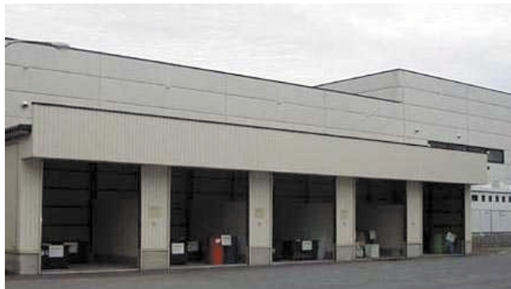
Waste storage facility (Tohoku Plant)
