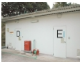
PCB storage building
