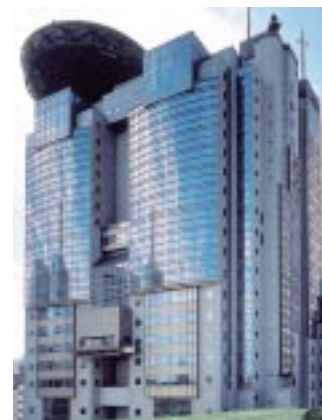
Tokyo Electron head office (TBS Broadcast Center 15 -18th Floor)
