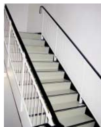
Newly installed handrail
